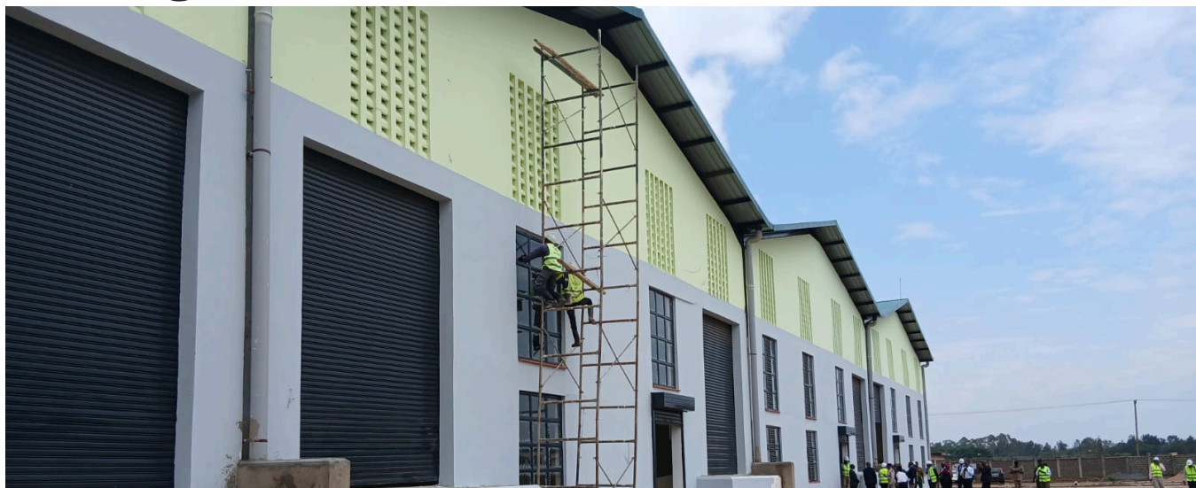
Kirinyaga County Aggregation and Industrial Park nears completion./Anne Sabuni
