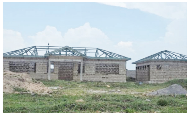
Figure 57: Administration and ablution blocks under construction
