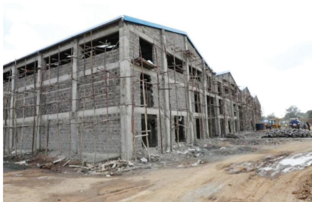
Figure 56: Superstructure works at the Aggregation warehouse
