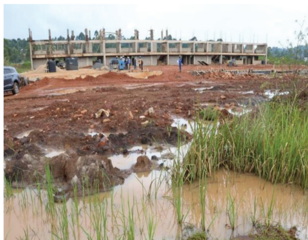
Figure 31: Aggregation, Cold Room and Storage units superstructure works - Nyamira County CAIP
