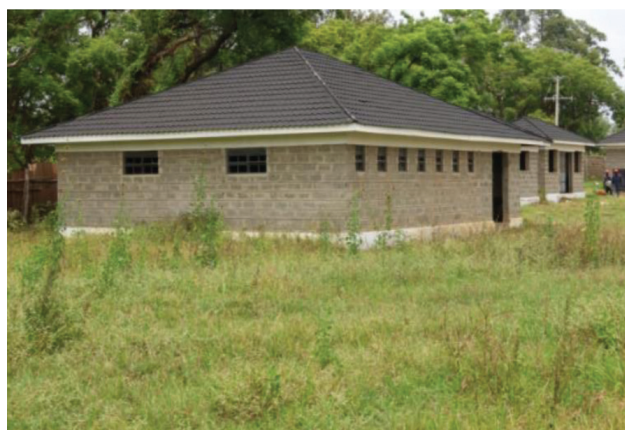
Figure 16: The Administration Block, Bungoma County CAIP
