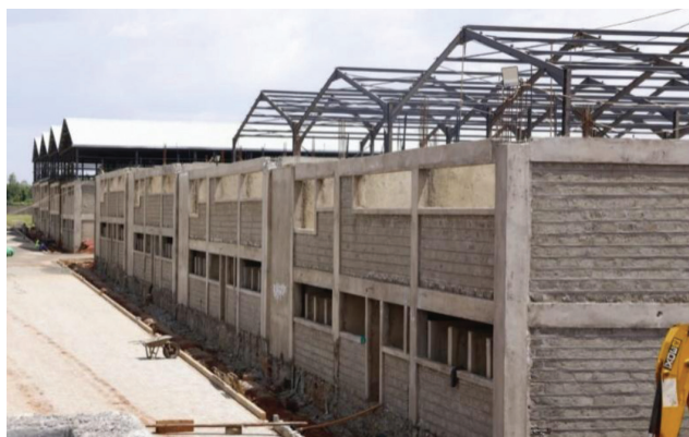
Figure 19: The sub & superstructures of value addition warehouse units - Busia County CAIP
