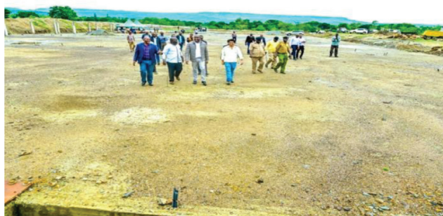
Figure 60: Foundation slab laid on the aggregation warehouse
