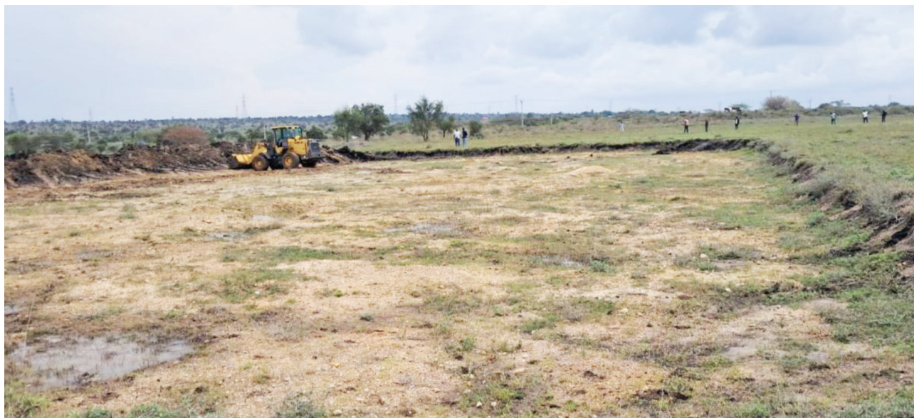
Figure 54: Site under Excavation
