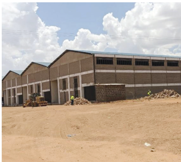
Figure 2: Aggregation warehouse (exterior)
