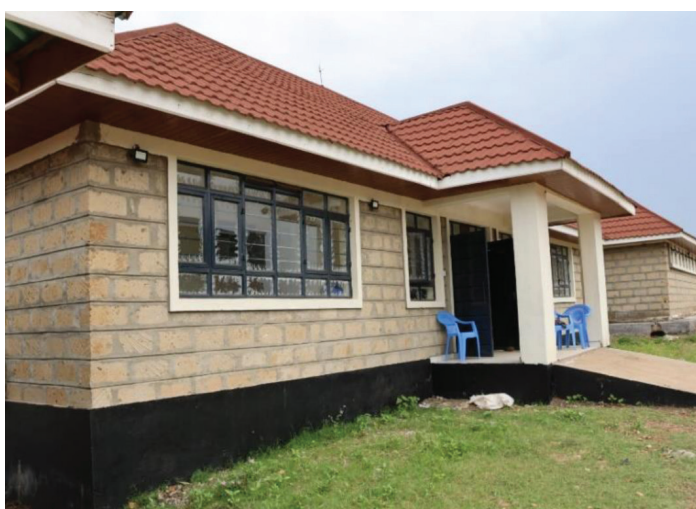
Figure 26: The Administration Block - Migori County CAIP
