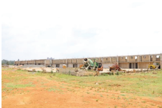
Figure 17: The ongoing works for the aggregation and value addition warehouses, Bungoma County CAIP
