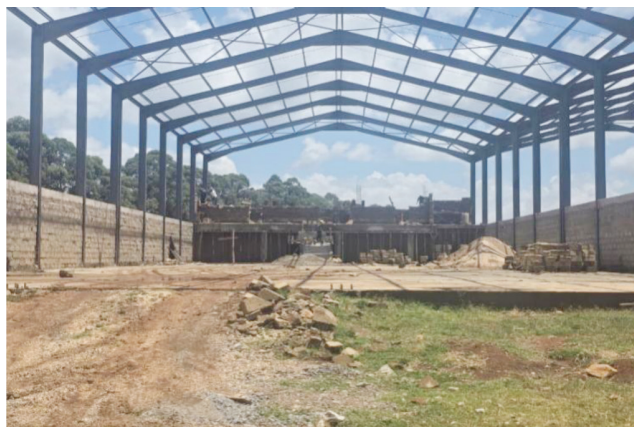
Figure 49: Value Addition warehouses superstructure under construction
