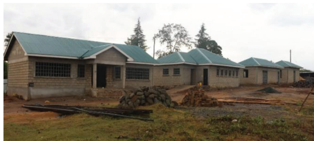
Figure 15: The Superstructure works for Pump and Power Houses, Kakamega County CAIP
