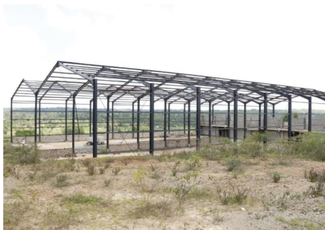
Figure 21: The Sub & Superstructures of Value Addition Warehouses, Siaya County CAIP
