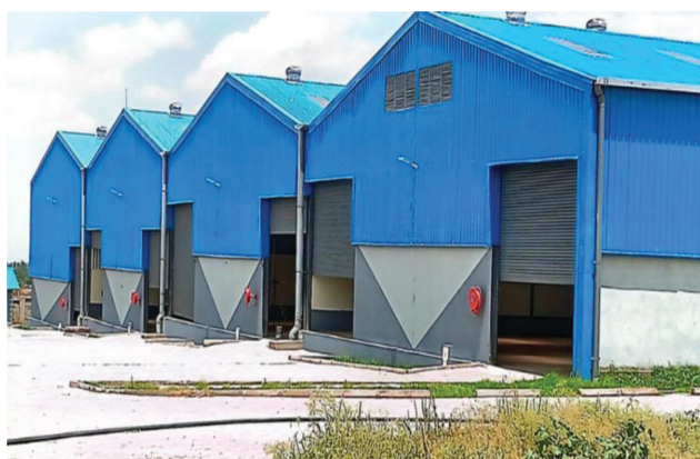
Aggregation and Value addition warehouses- MERU County CAIPs
