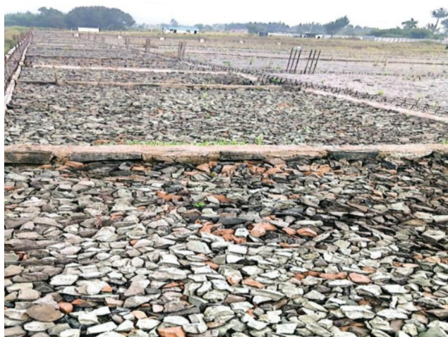
Figure 34: Slab for the Value Addition block, Nyandarua CAIPs
