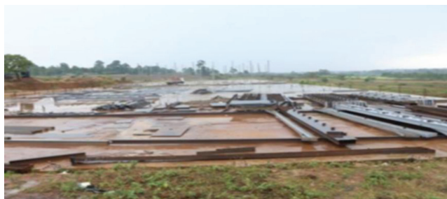
Figure 14: Substructure works for Aggregation, value addition warehouses and cold rooms, Kakamega County CAIP
