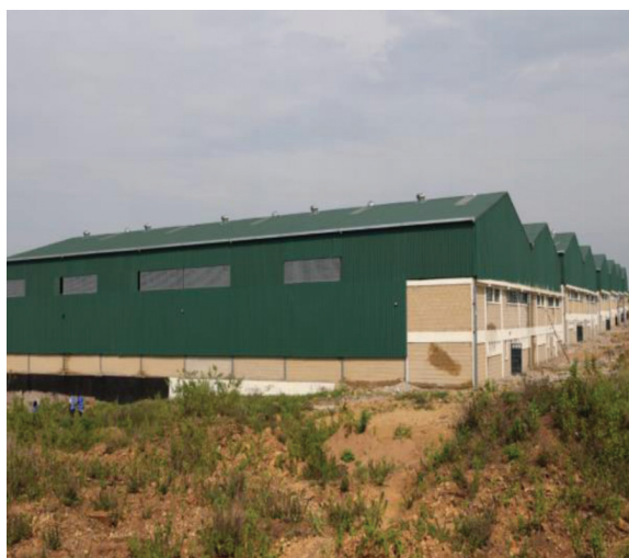
Figure 27: The Aggregation, Cold Room and Storage units - Migori County CAIP
