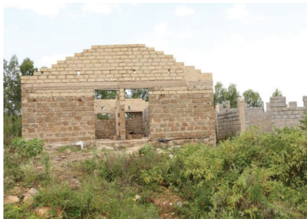
Figure 20: The Administration Block works, Siaya County CAIP
