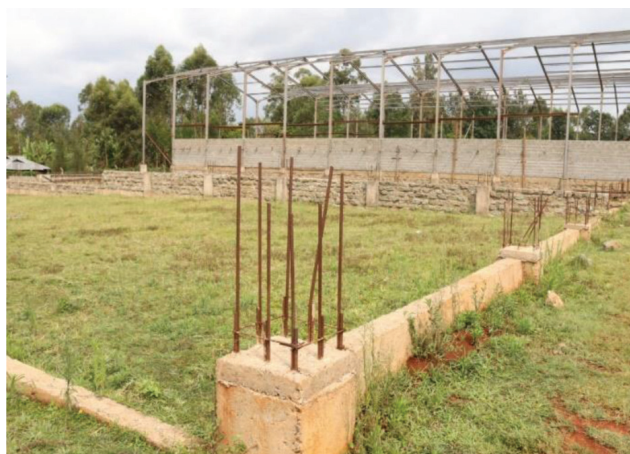
Figure 23: The Superstructure works , Vihiga County CAIP
