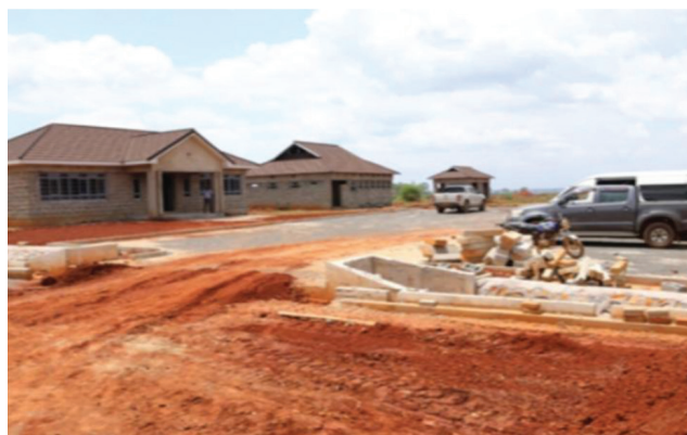
Figure 18: ongoing works on Administration Block & Ablution units - Busia County CAIP
