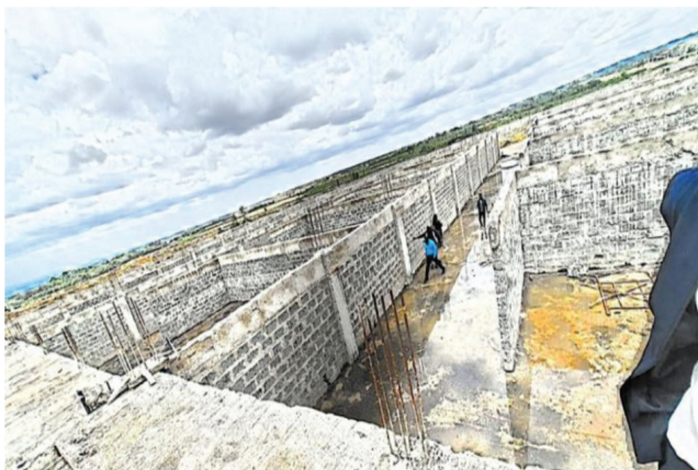
Figure 36: Aggregation and Value Addition warehouse wall structure
