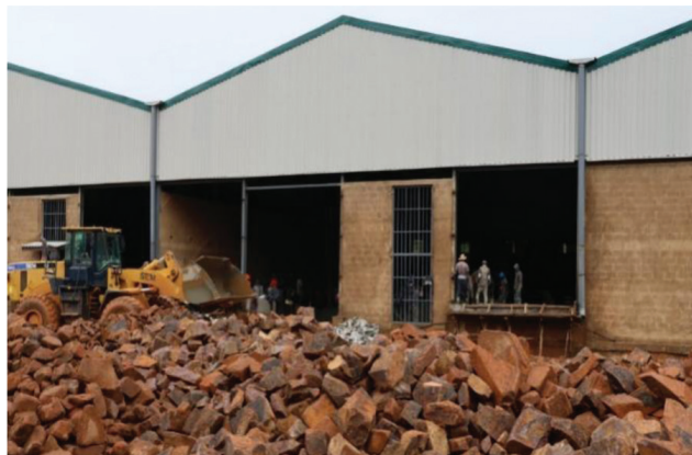
Figure 29: The Value Addition warehouses - Kisii County CAIP
