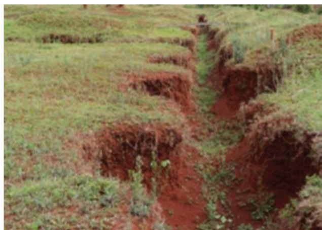
Figure 22: The excavations for walling and column bases works for Aggregation Warehouses , Vihiga
