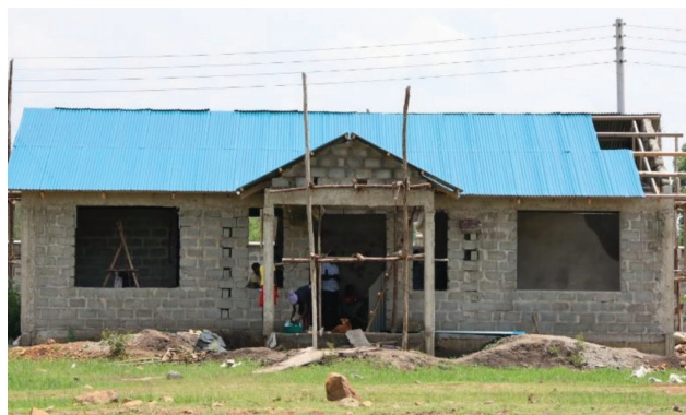
Figure 25: The ongoing works on Administration Block - Homa Bay County CAIP
