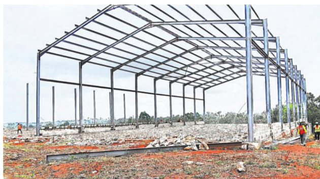
Figure 39: Steel structure for aggregation-Murang'a CAIPs
