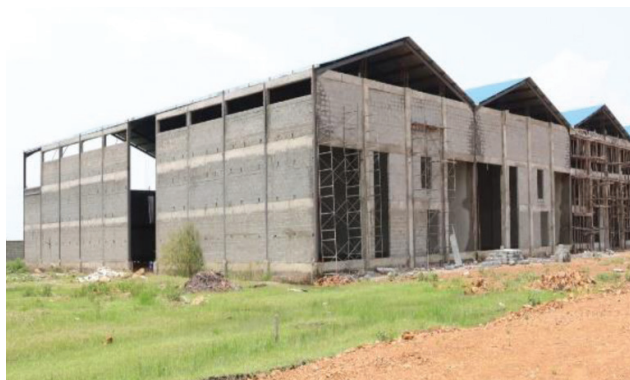
Figure 24: The Aggregation and Value addition warehouse superstructure works - Homa Bay County
