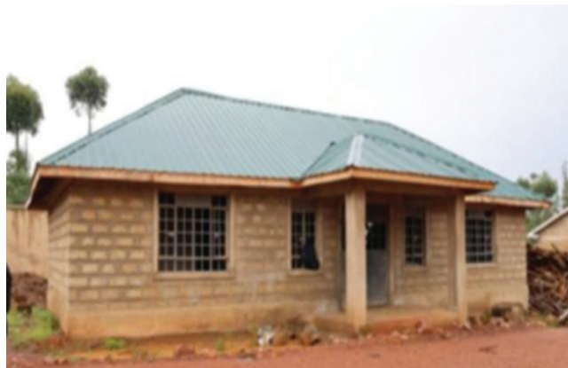
Figure 28: The Administration Block - Kisii County CAIP
