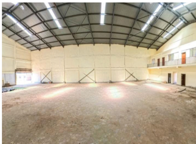
Figure 62: Value Addition warehouse (interior)
