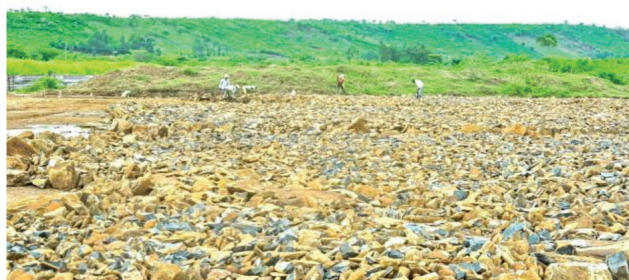
Figure 59: Hand packing of the foundation for the value addition warehouse
